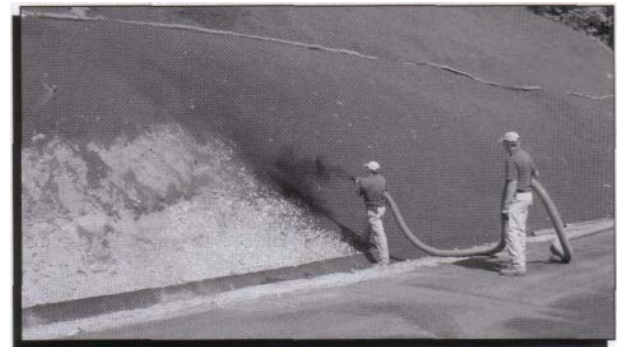
The contractor used a pneumatic blower to apply the compost.
