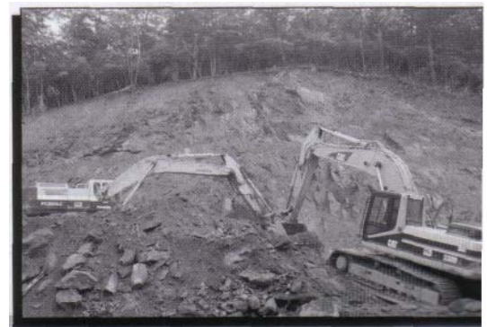
Trackhoes work together to excavate the slope down to established grades.
